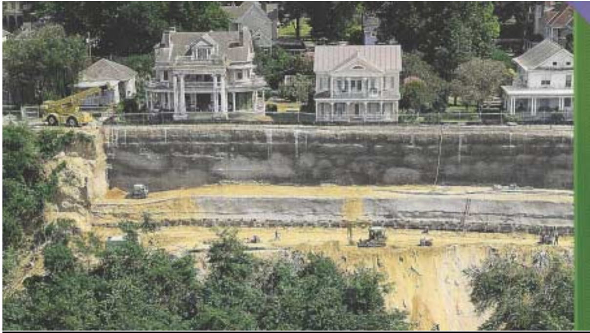
Photograph 5. High capacity SBMAs in difficult "loess" soils in Natchez, MS.
